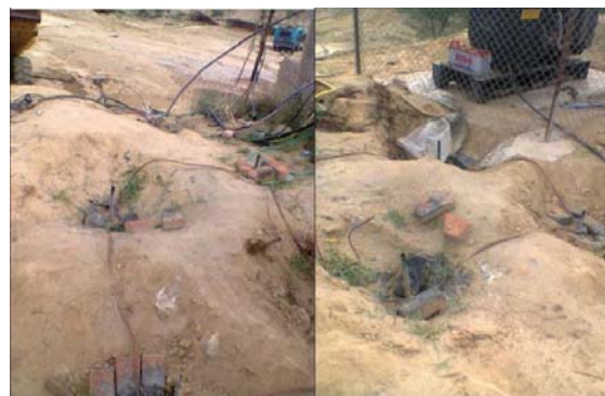
Figure 2: Implementation of grounding channel by combining four portable grounding blocks of dimension 10" x 10" x 14"
