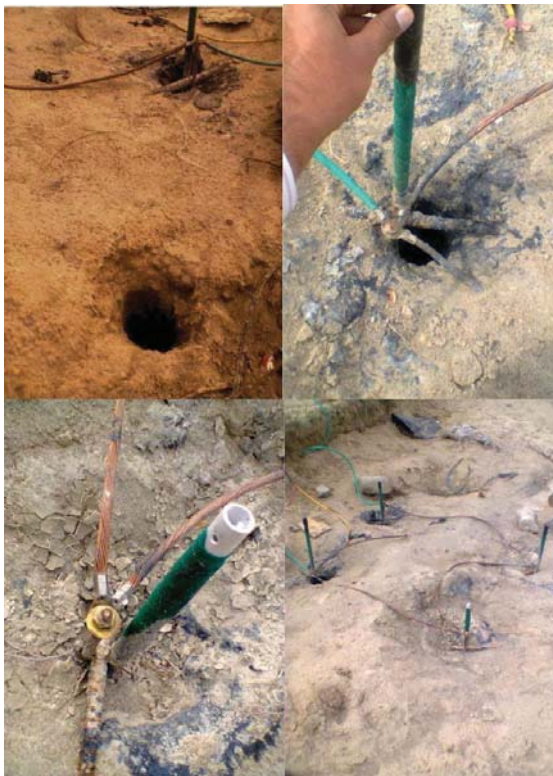
Figure 3: Implementation of grounding channel using rod method
