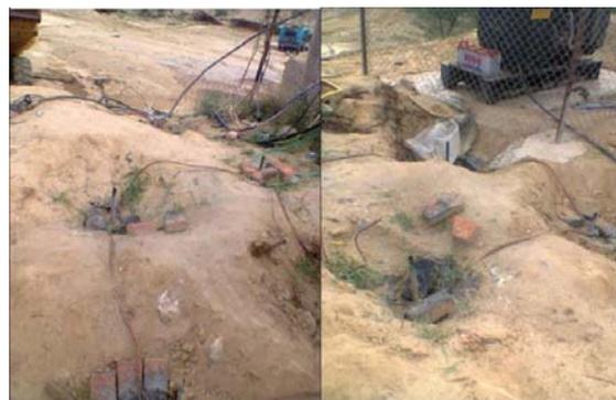
Figure 2: Implementation of grounding channel by combining four portable grounding blocks of dimension 10" x 10" x 14"
