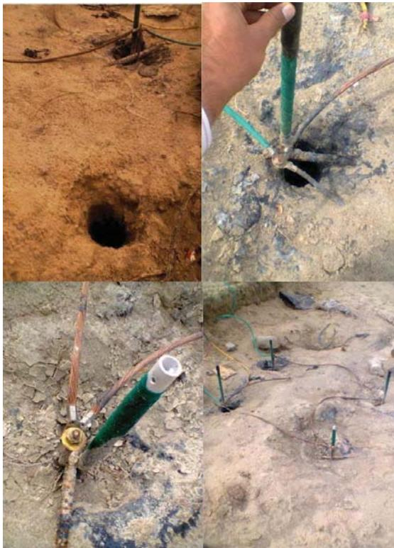
Figure 3: Implementation of grounding channel using rod method
